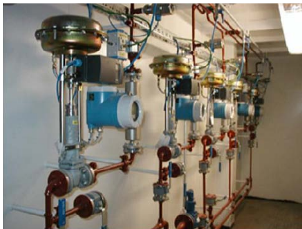
Figure 6.28: Measuring and dosing station with pneumatic valves
