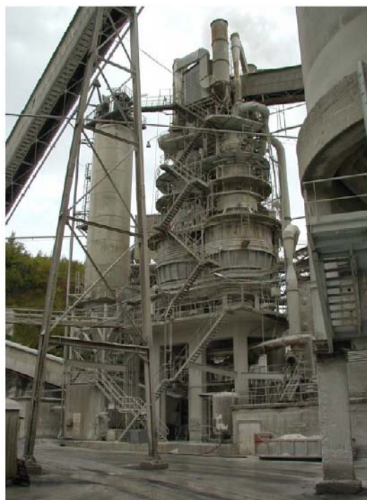
Figure 2.23: Example of a PFRK Source: [44, EuLA, 2006]
