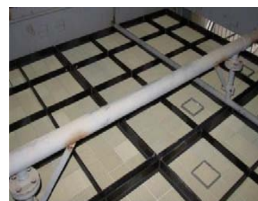
Figure 1.68: Example of a module position used for the SCR technique
