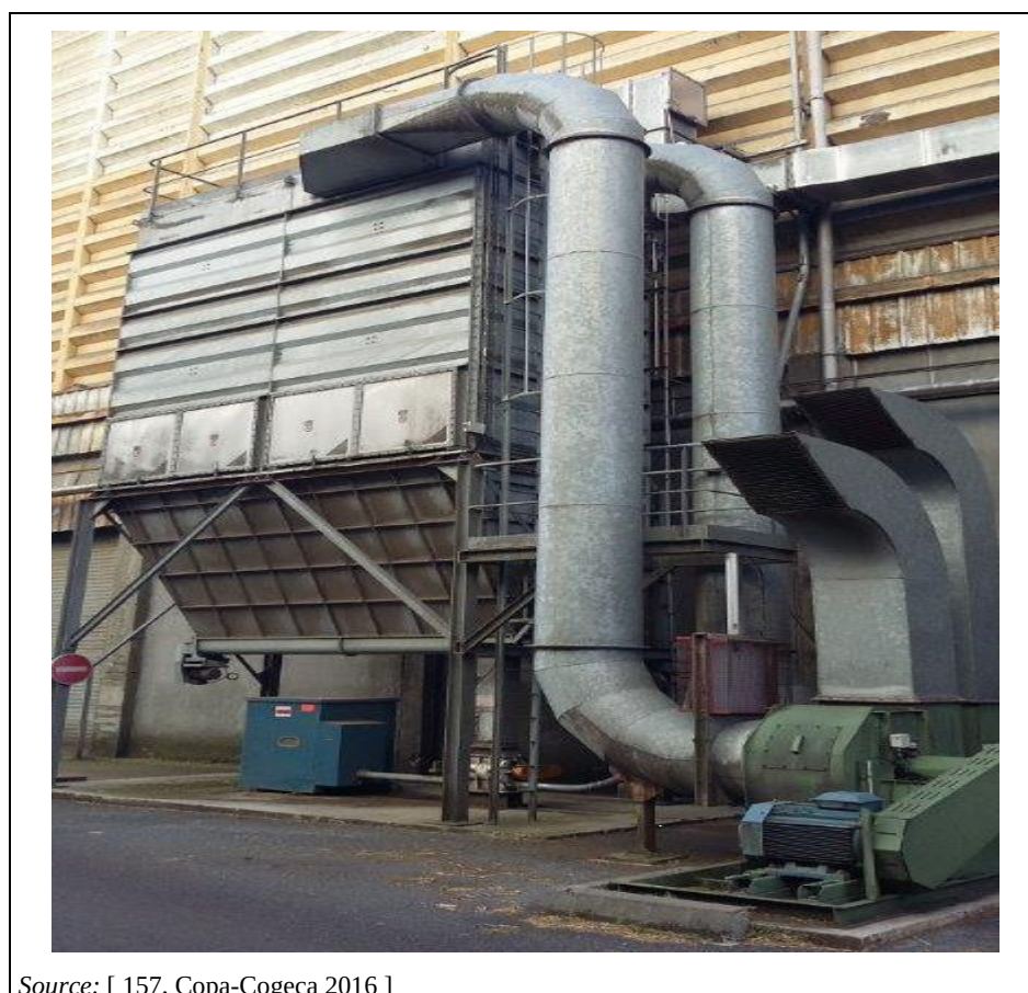
Figure 2.43: Picture of an industrial bag filter
