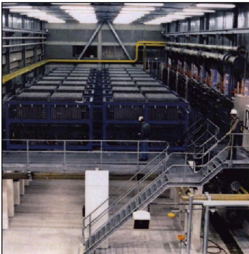
Figure 2.10: View of a membrane cell room equipped with bipolar electrolyzers (Source: Hoechst-Uhde)
